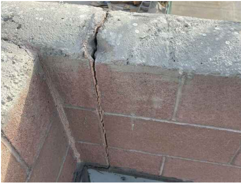
vertical cracks through out parapet wall and coping
