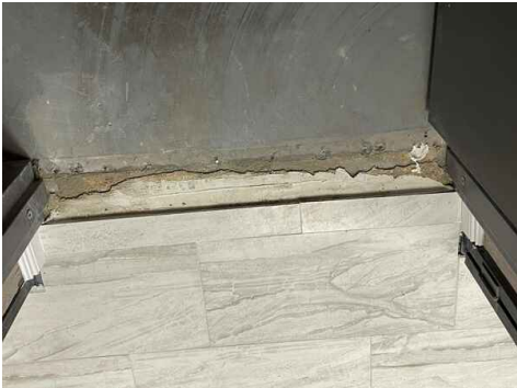
Threshold deteriorating
