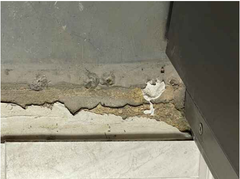
Threshold deteriorating
