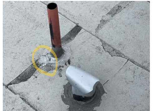
Boot over ventilation is old and cracking, will allow water intrusion if not taken care of.
