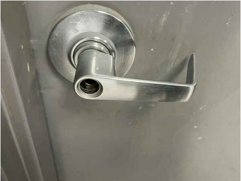
Hardware on doorknob damaged, door still opens
