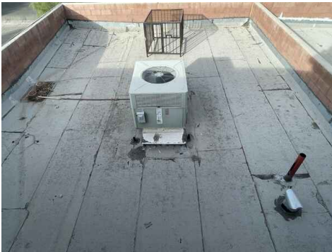
rust on ventilation, debris blocking drain causes ponding
