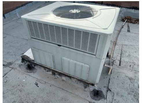
Boot over ventilation is old and cracking, will allow water intrusion if not taken care of.
