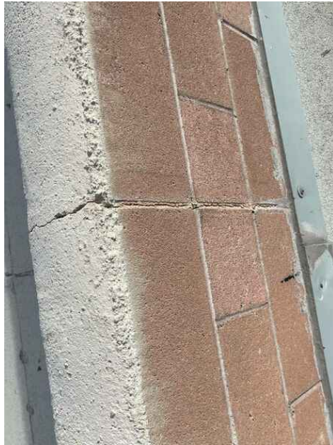
cracks on parapet walls and coping
