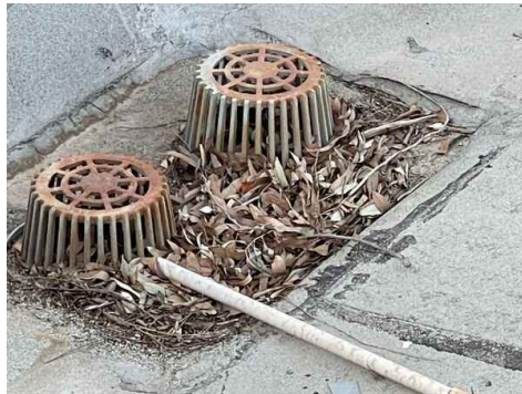
roof drain covered with debris causes ponding, and water intrusions through out roof.
